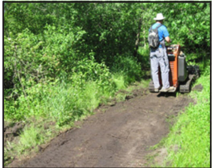
Mike from Trail Design Specialists working with a Ditch Witch - specialized trail equipment. The tread was raised almost 6 inches using soil from the park, topped with gravel and compacted. The stumps were grubbed for a smooth hiking surface and the trail will no longer puddle water.
